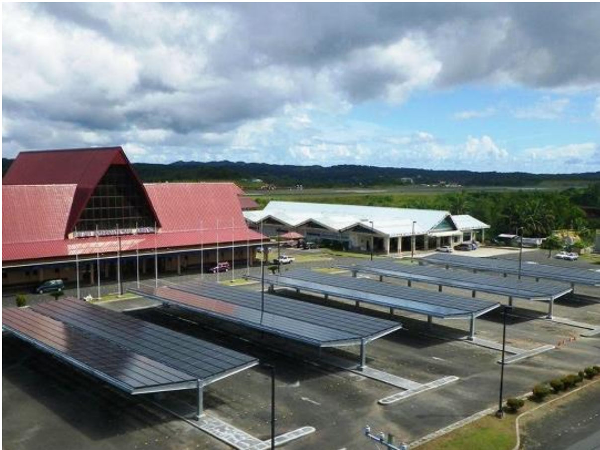
Figure 16: The solar array installed at the airport carport (Palau).
